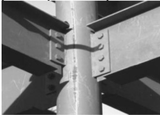
a) Typical Fin Plate Connection
