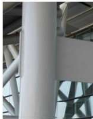
b) Typical Through plate Connection
